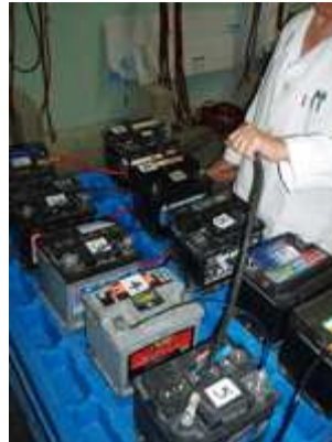
Connecting the batteries
